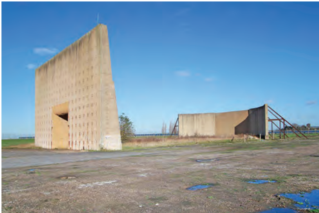
The first blast wall at K2 is 12 metres high. There is a rectangular aperture in the centre of the wall to allow the exhaust plume from the test to pass through to the second lower blast wall
